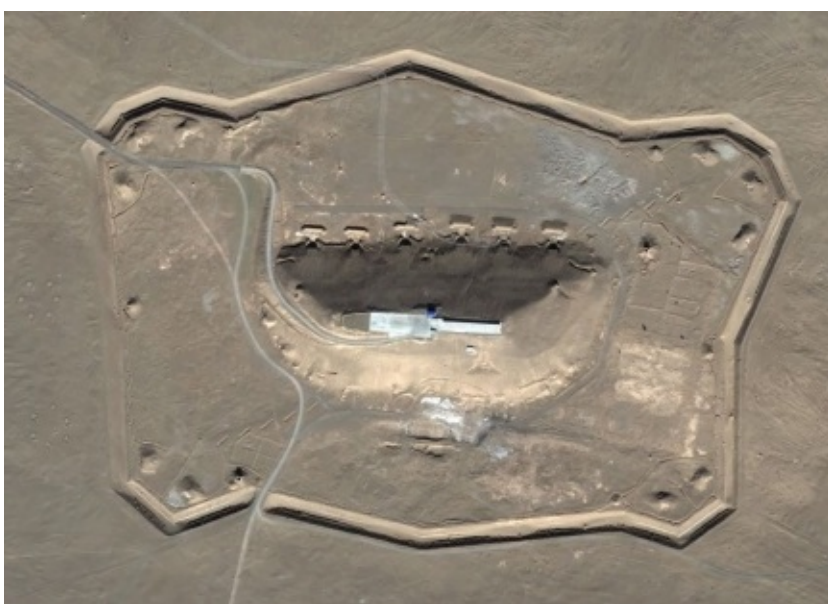
Figure 31. Bunker facility with underground tunnels linked to Dingxin Test and Training Base
